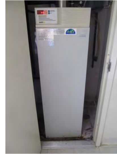
Each unit is equipped with a combination hydronic boiler/domestic hot water generator – Equipment is serviceable but at or near end of expected useful service life
