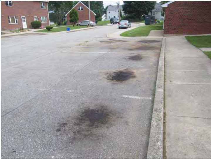
Asphalt-paved parking surfaces exhibit wear and automotive fluid staining
