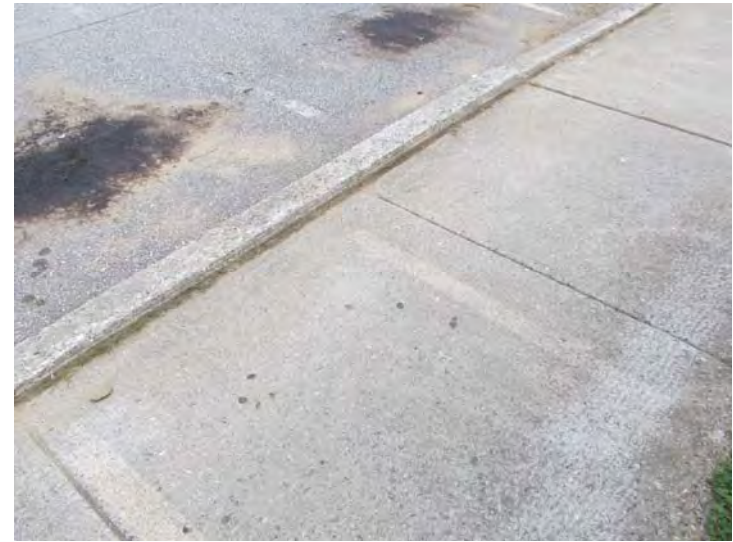
Concrete sidewalks vary in condition – Note subsidence along curb edge posing possible trip hazard
