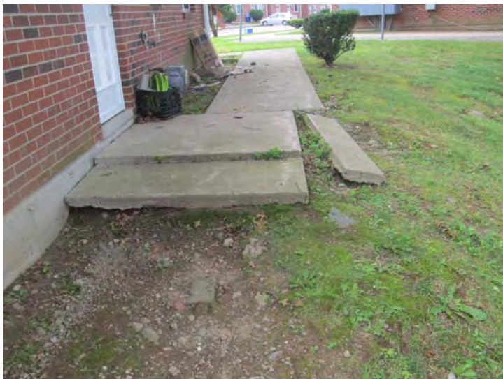
Drainage improvements needed to help reduce erosion
