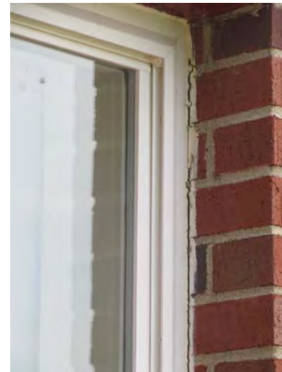
Perimeter caulking at windows exhibits shrinkage at some locations
